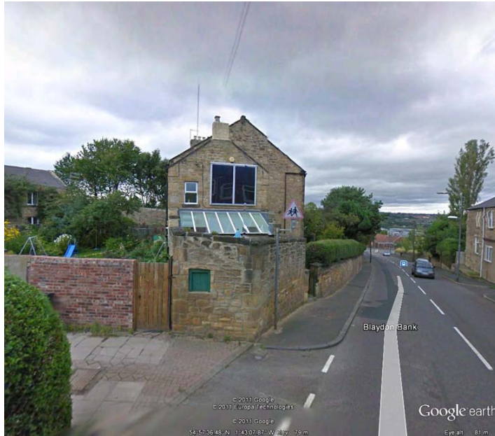
Figure 2 Photovoltaic cells on the elevation of a house in urban Blaydon-upon-Tyne, Gateshead, Tyne and Wear
